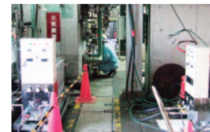
Geothermal plant turbine oil (SRC-8110-162V/816-22V)
