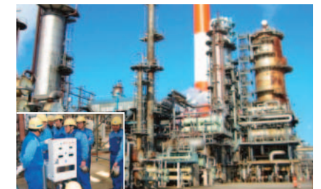
Refinery turbine lubricating oil (SRC-814-15V; explosion proof)
